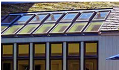
EDM – Metal roof flashing Flashing pieces interlock with roofing material for a weather tight installation.
